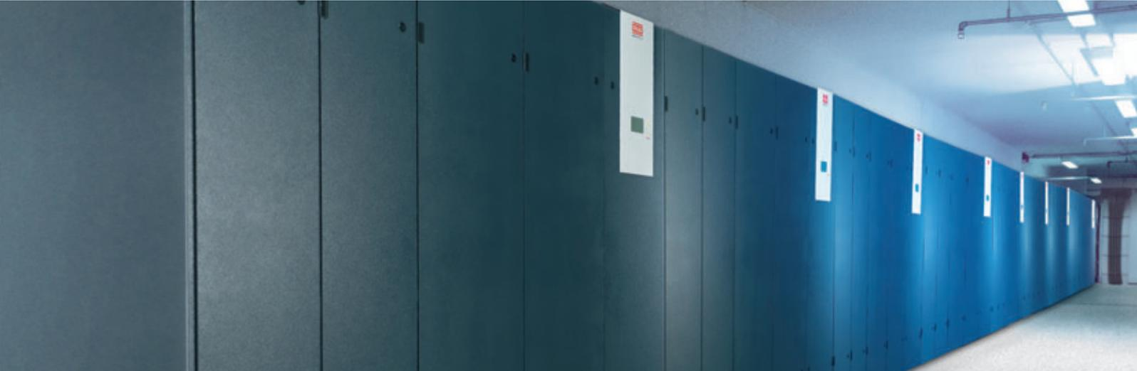
STULZ CyberAir 2 allows for both central and distributed arrangement of A/C units. Every unit has its own intelligence. Up to 20 units work together in the system network.
